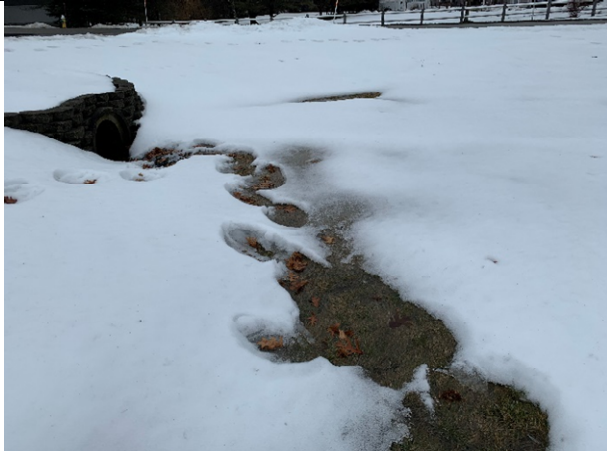
29 Gundalow - 1 (Drainage Area)
