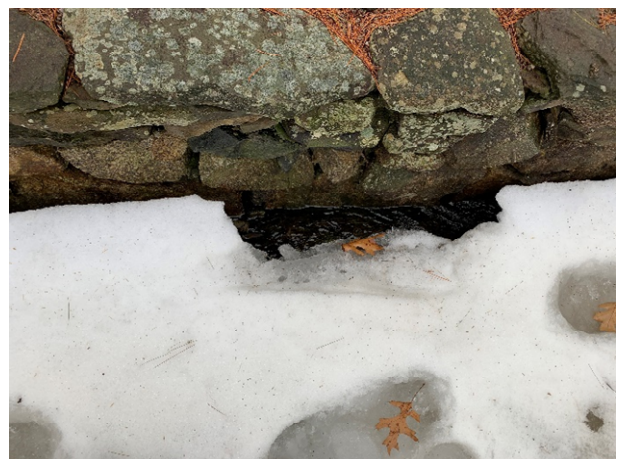
4 Brickyard Circle - 2 (Drainage Course)
